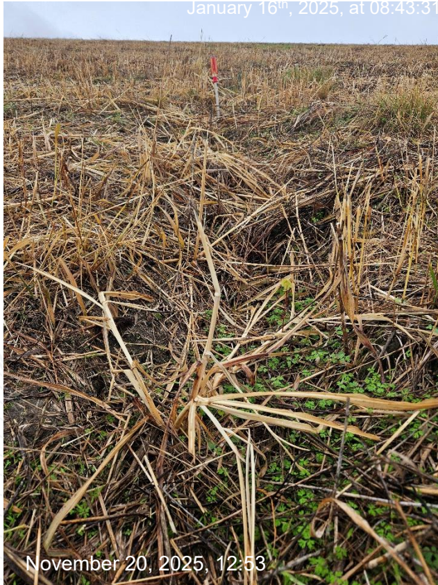
Erosion on the W side of impoundment cap. Photo taken facing east towards the impoundment cap. Approx. 4-6" deep.
