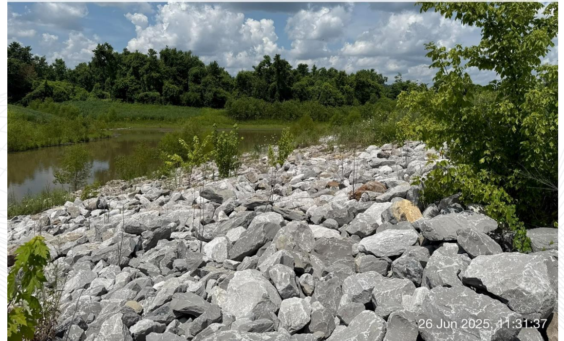
Woody vegetation on south-facing riprap. Picture facing west from riprap.
