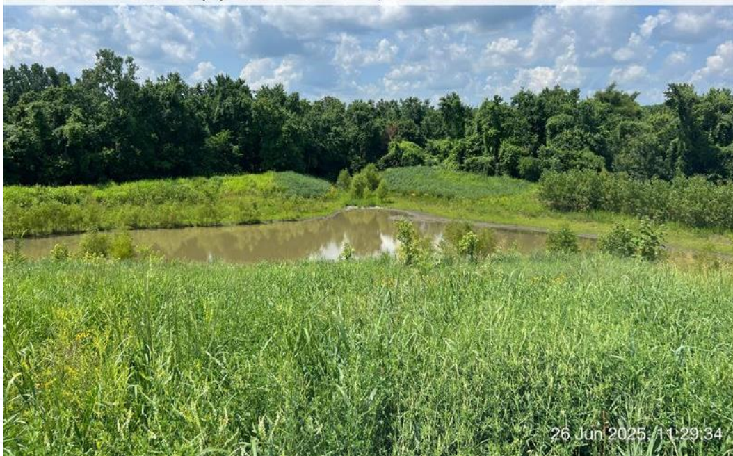
Ponded area in southwest corner of site as viewed from atop impoundment cap.
