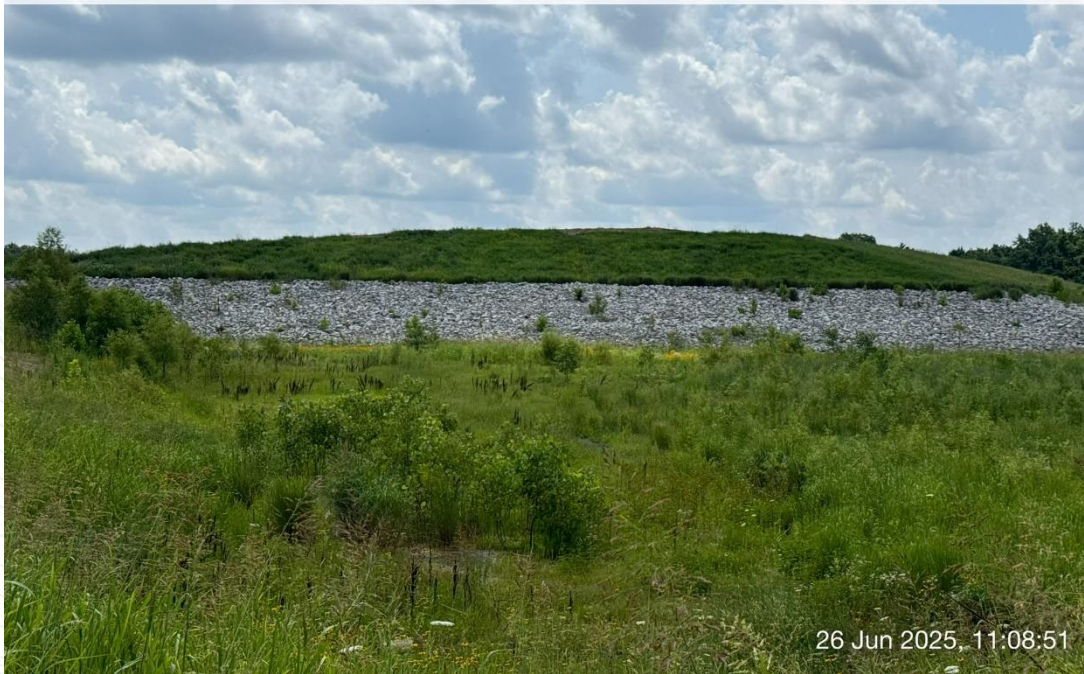
Woody vegetation on north-facing riprap. Picture facing south from path north of the impoundment.
