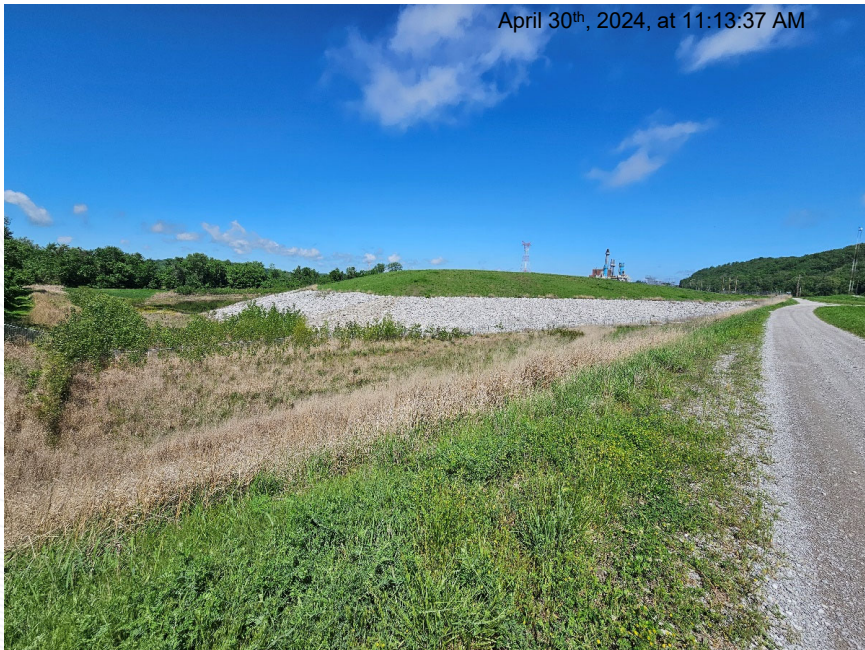
Facing north along the repaired fence-line, riprap, and levee area.
