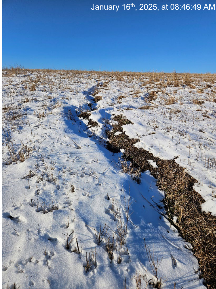
Erosion on the west side, roughly 6" deep, of impoundment cap. Photo taken facing east from the bottom of the impoundment cap.
