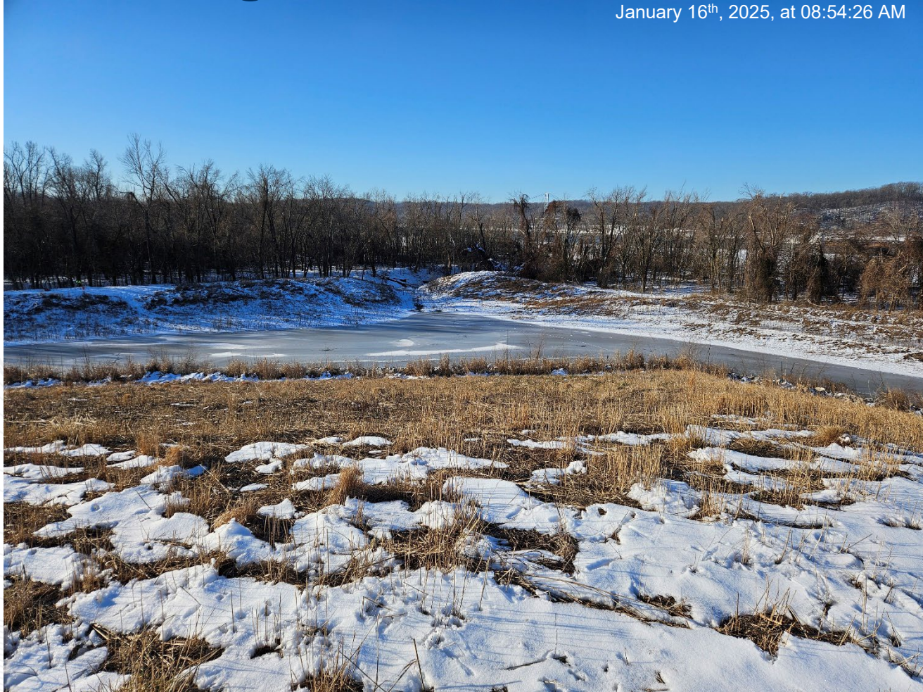
Ponded area in southwest corner of site as viewed from atop impoundment cap.
