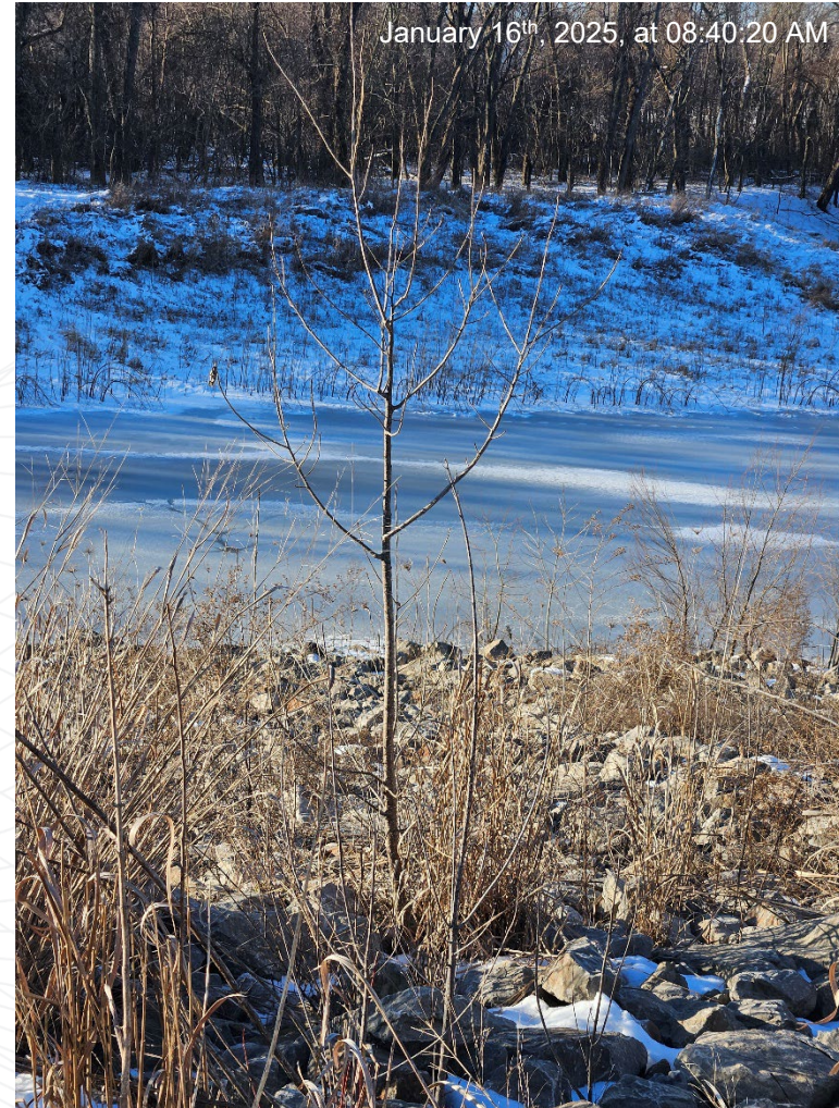
Woody vegetation on south facing riprap. Picture facing south from atop impoundment cap.
