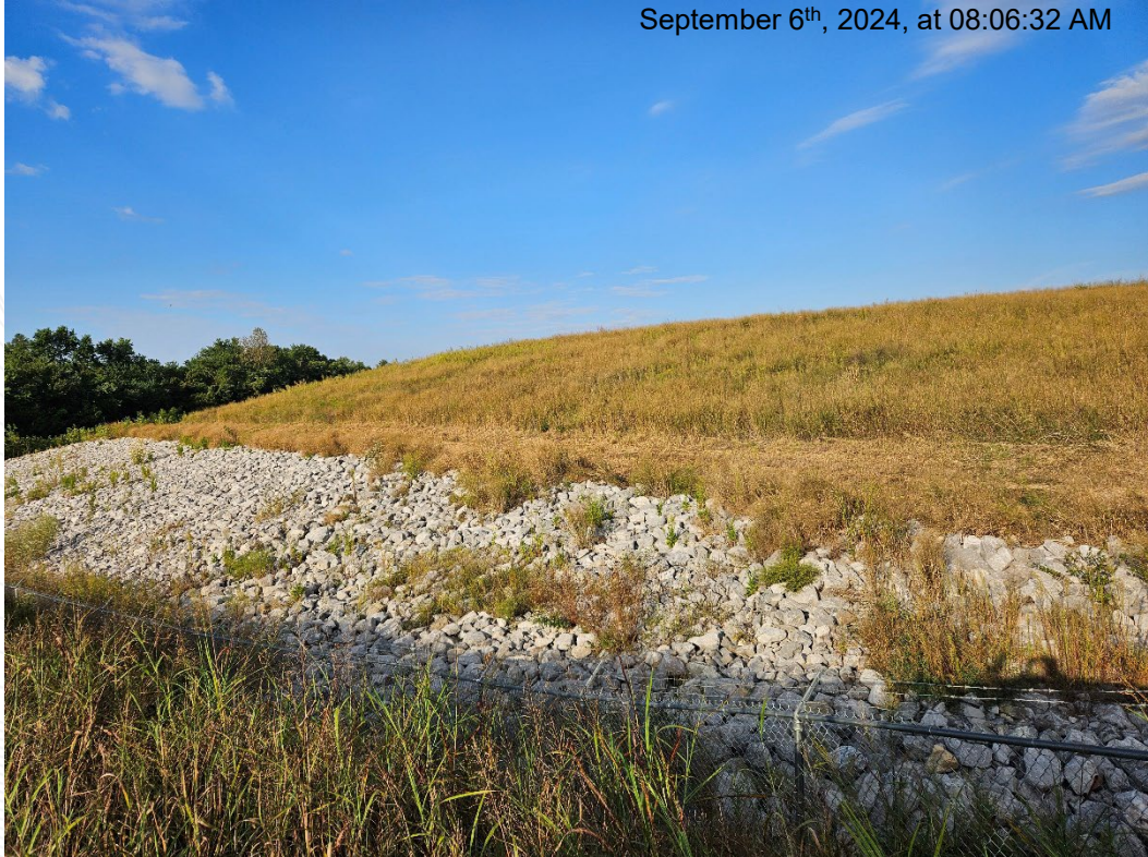
Facing west along the repaired fence-line, riprap, and levee area.
