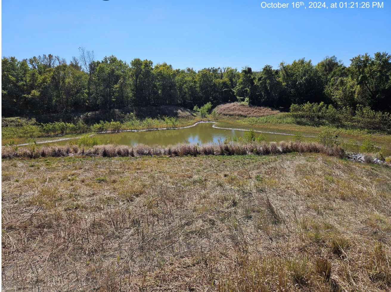
Ponded area in southwest corner of site as viewed from mowed impoundment cap. Potential woody vegetation removal in spillway will be assessed in Q1 2025.
