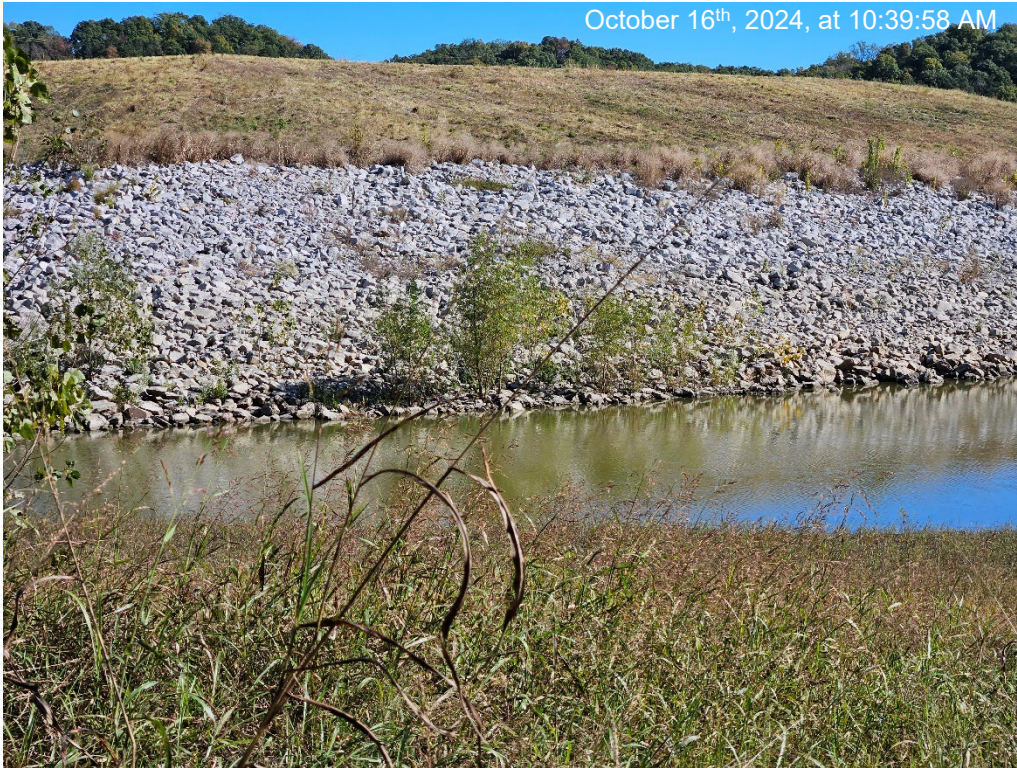
Sparse woody vegetation on southern riprap
