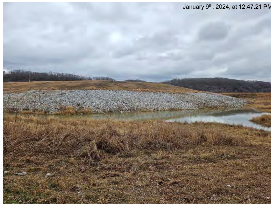
Ponded area in southwest corner of site and impoundment cap as viewed from southwest corner.
