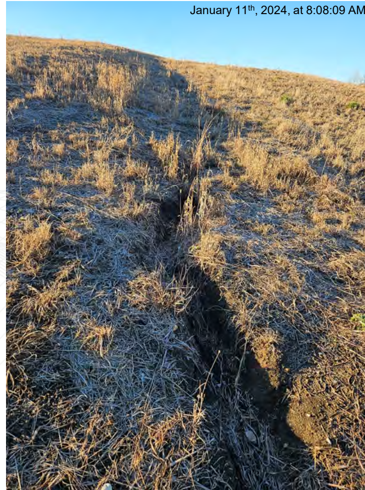
Erosion from western side of impoundment cap.
