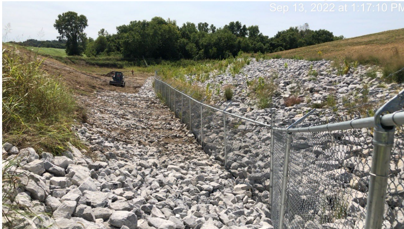
Facing south along recently repaired fenceline area.
