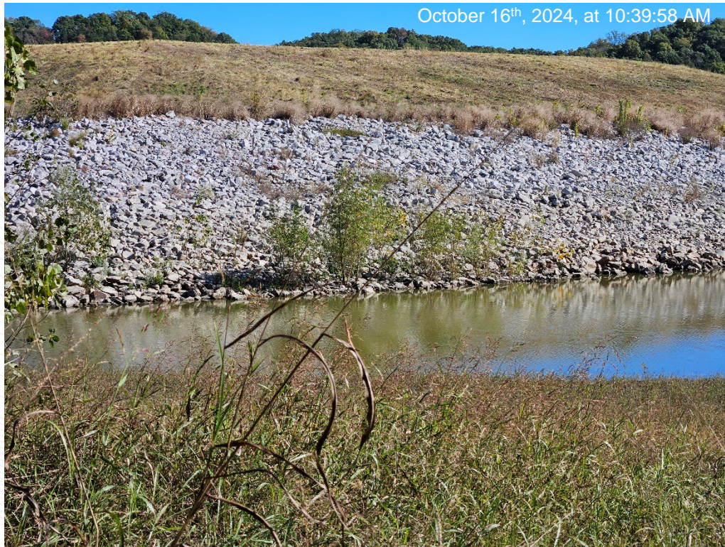
Sparse woody vegetation on southern riprap
