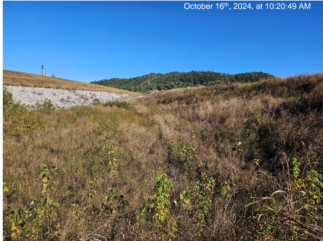
View facing north along the fence-line, riprap, and levee area.
