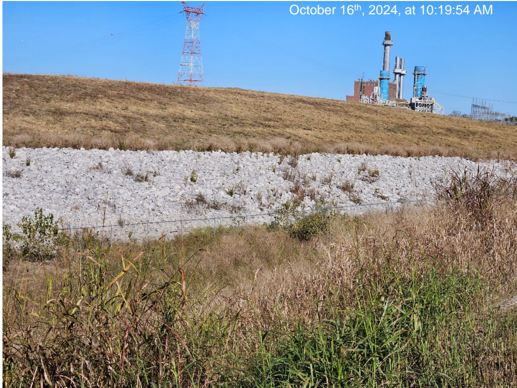
View facing northwest along the fence-line, riprap, and levee area.
