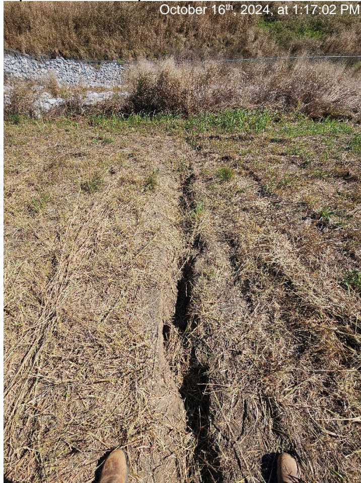
Erosion on the west side, roughly 6" deep, of impoundment cap. Photo taken facing west from the top of the impoundment cap.
