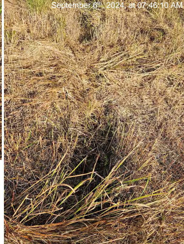
Erosion channel on south side of impoundment cap.
