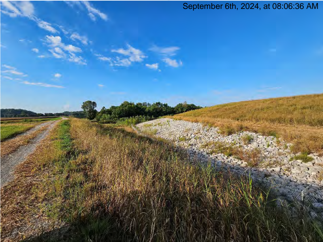
Facing south along the repaired fence-line, riprap, and levee area.
