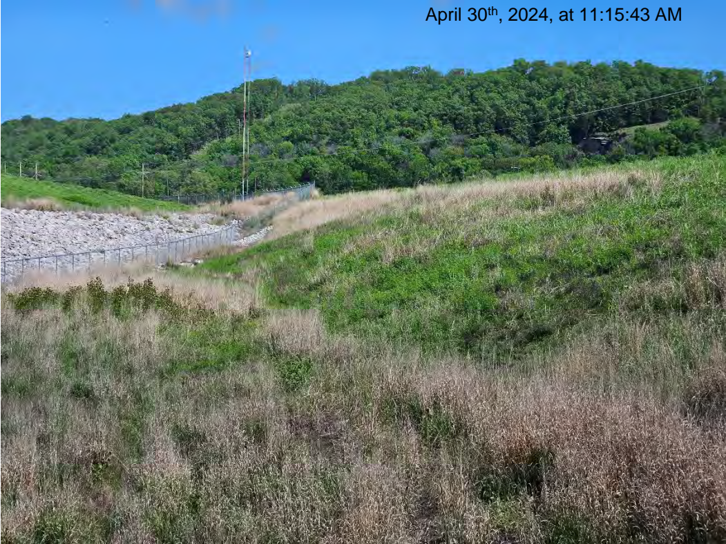
Facing northeast along the repaired fence-line, riprap, and levee area.
