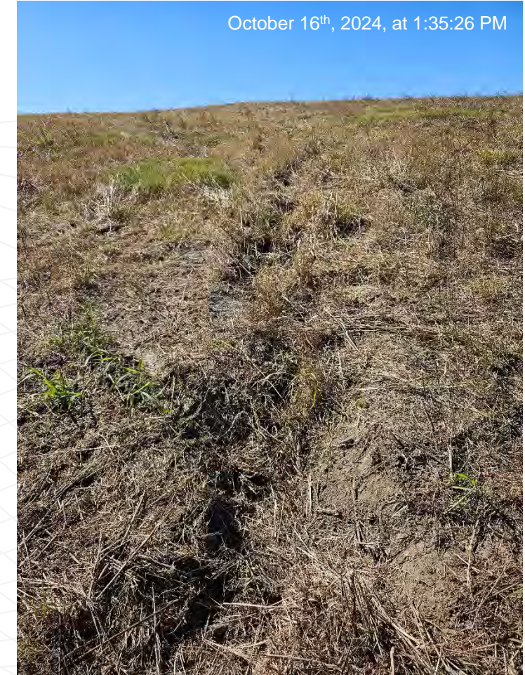
Erosion on the east side of impoundment cap. Photo taken facing west from the bottom of the impoundment cap.
