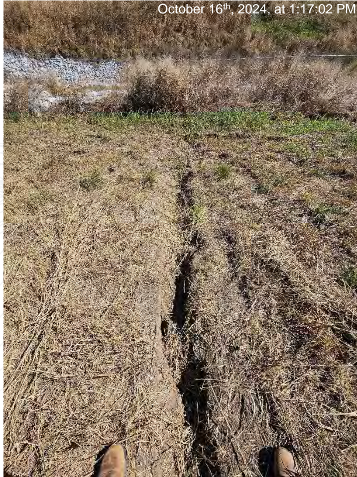
Erosion on the west side of impoundment cap. Photo taken facing west from the top of the impoundment cap.
