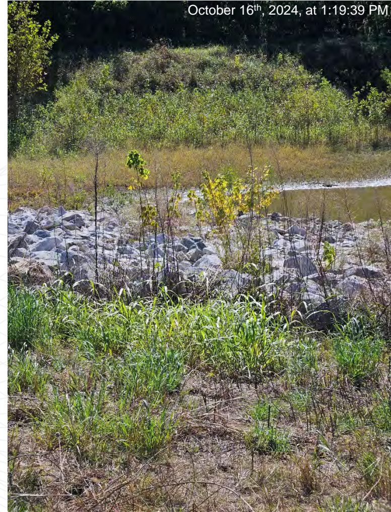
Woody vegetation on south facing riprap. Picture facing south from atop impoundment cap.
