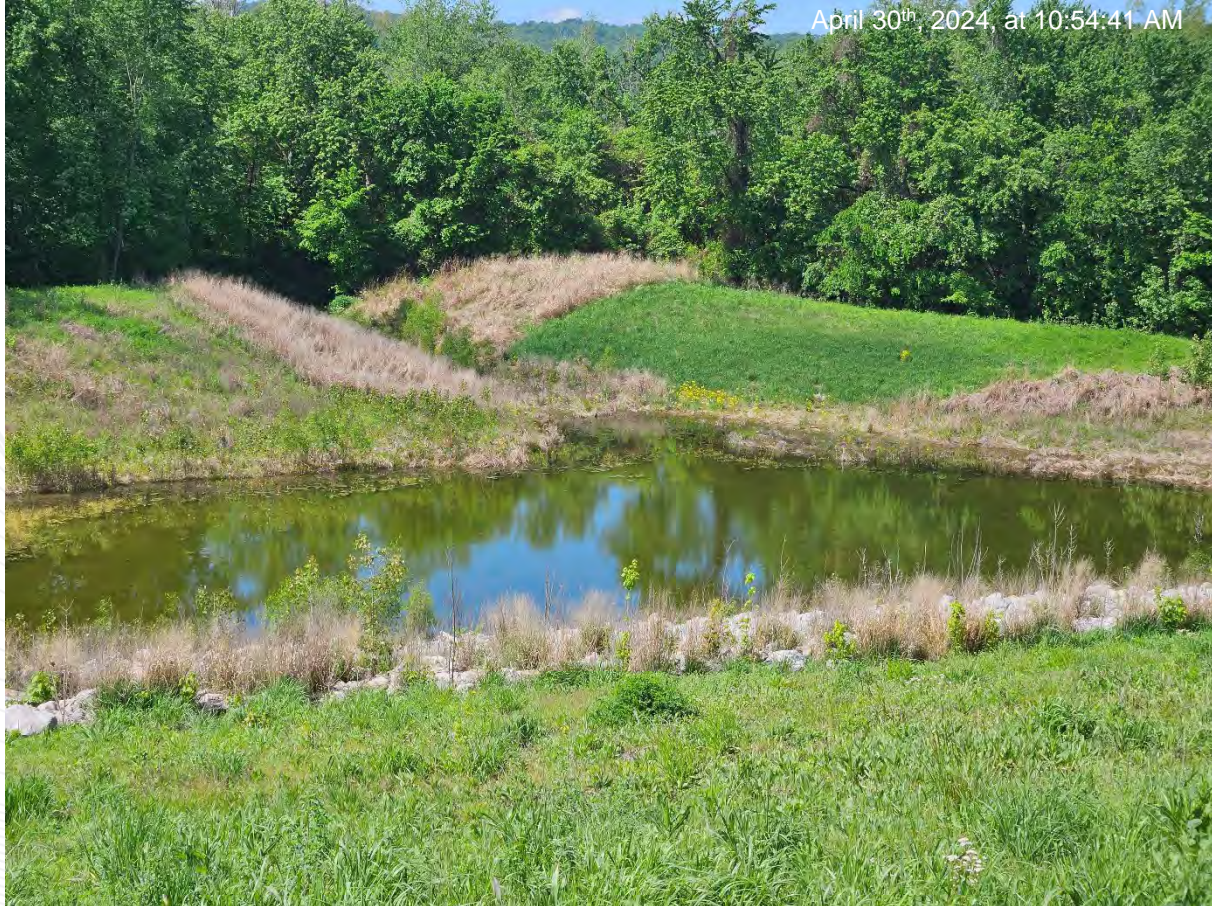
Ponded area in southwest corner of site as viewed from mowed impoundment cap.
