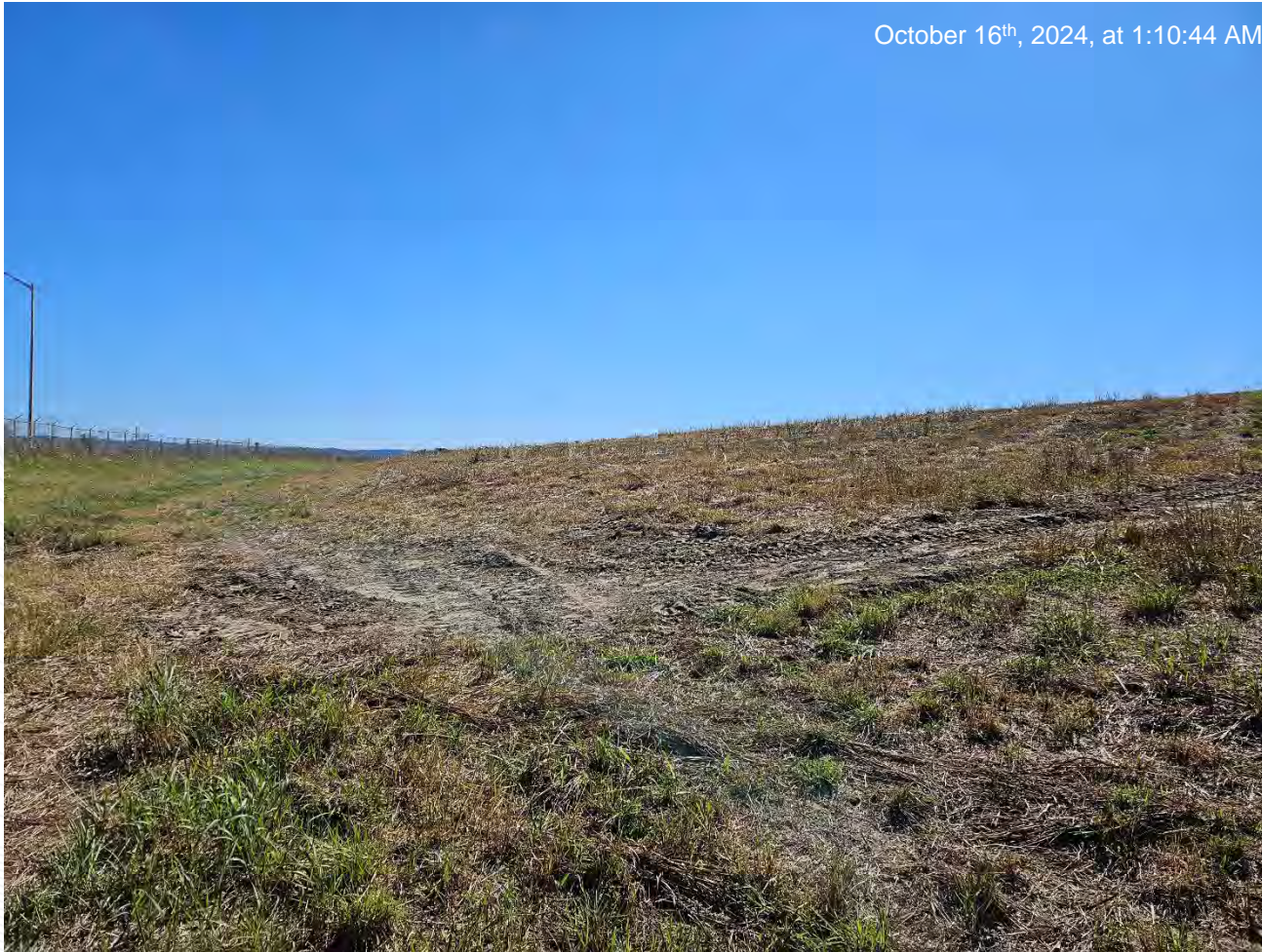
Erosion repairs made near the northeastern section of the impoundment cap. Photo taken from northeastern section of impoundment cap, facing south.
