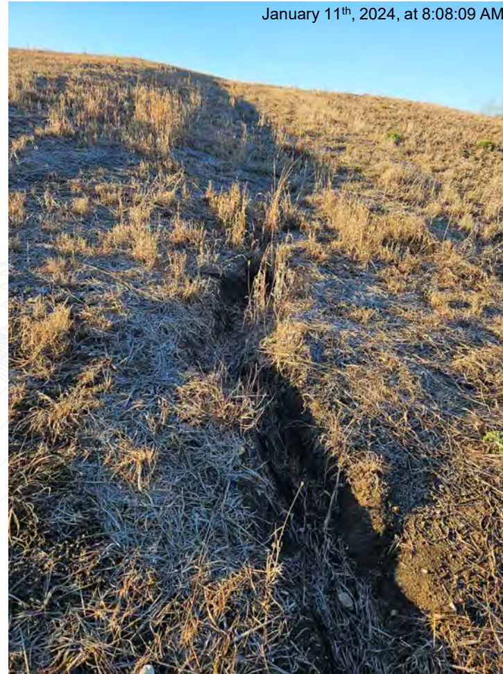
Erosion from western side of impoundment cap.
