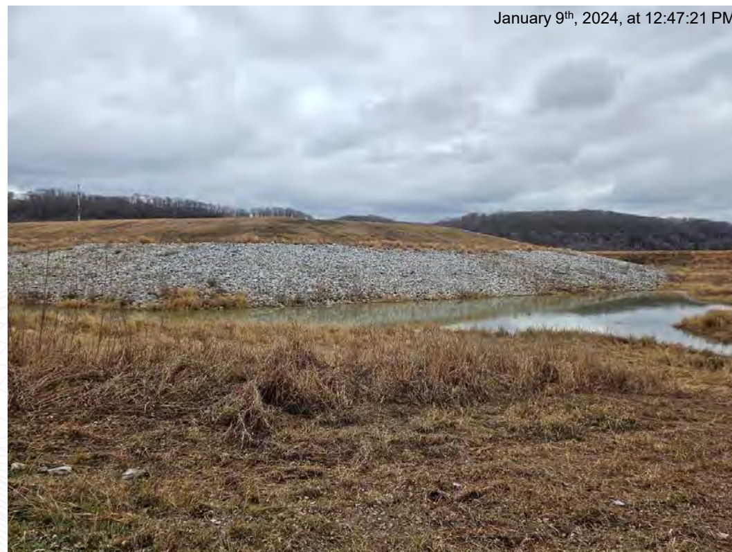
Ponded area in southwest corner of site and impoundment cap as viewed from southwest corner.
