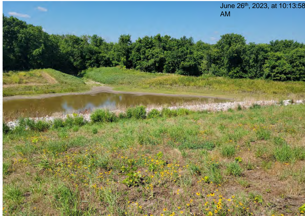
Ponded area in southwest corner of site as viewed from mowed impoundment cap.
