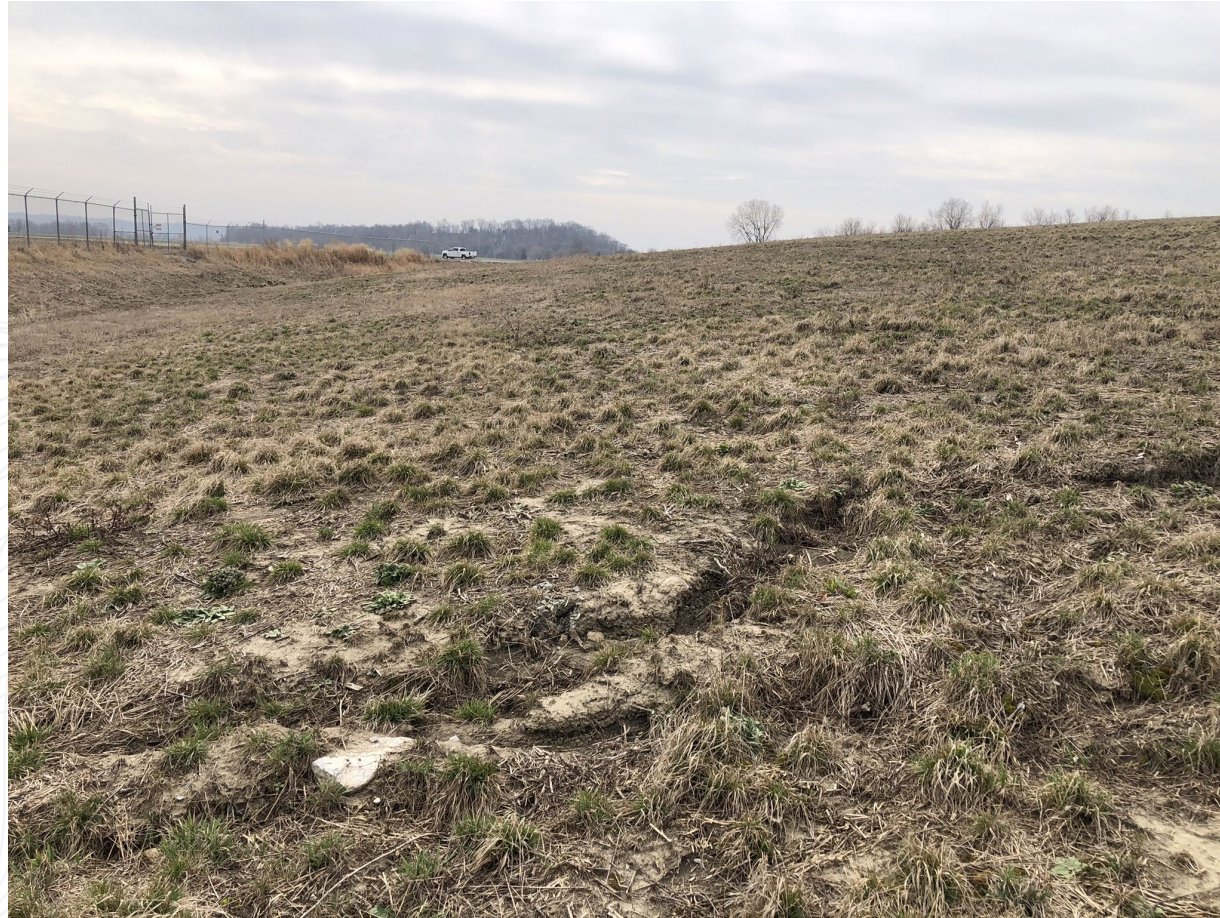
Facing south on east side of impoundment cap.
