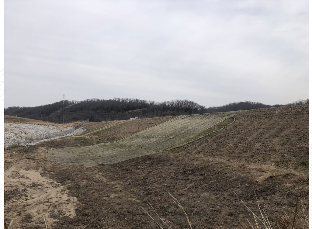
Facing northeast towards repaired section of USACE levee.
