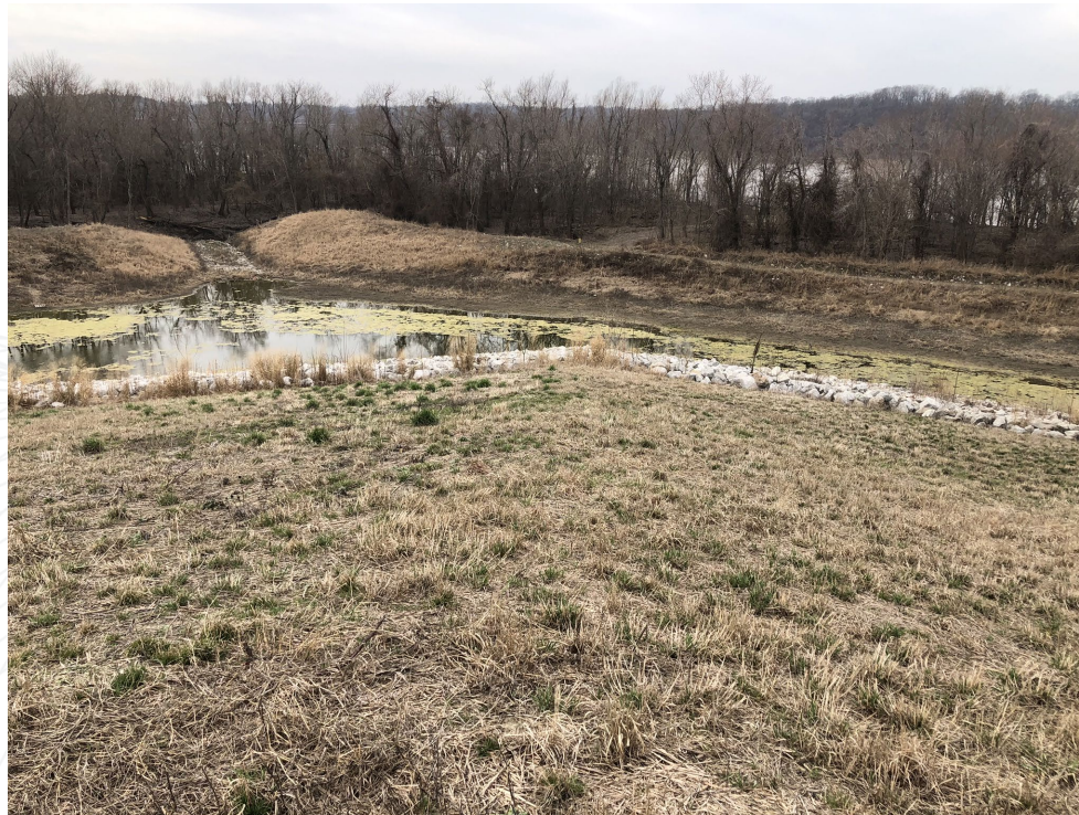
Ponded area in southwest corner of site as viewed from impoundment cap.
