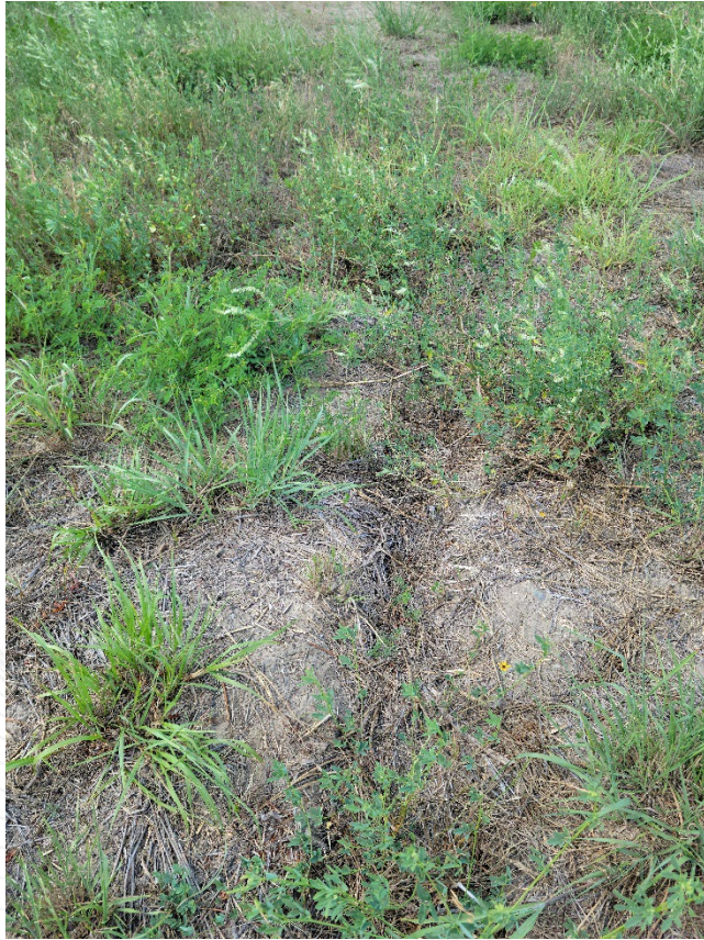
Erosion up to 9" deep - facing east from center-east side of impoundment cap.
