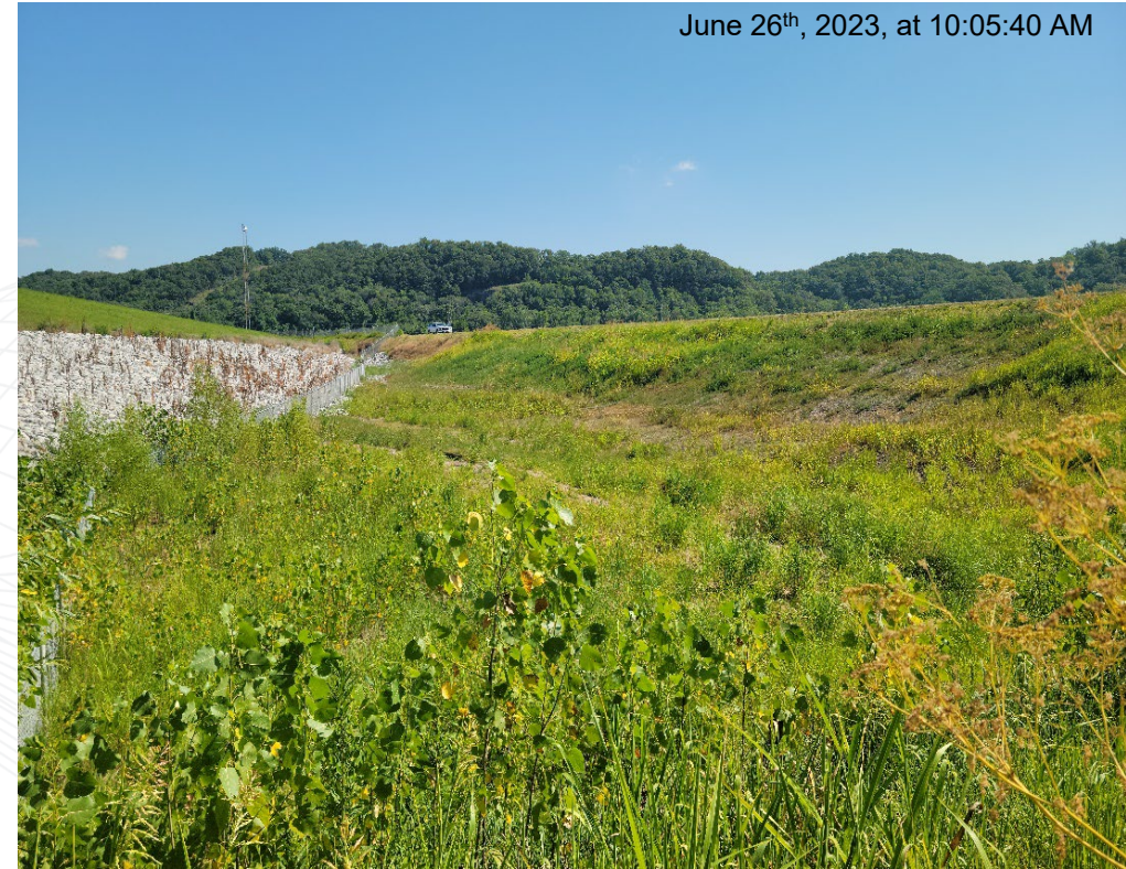
Facing northeast towards repaired section of USACE and GTEC levee sections.
