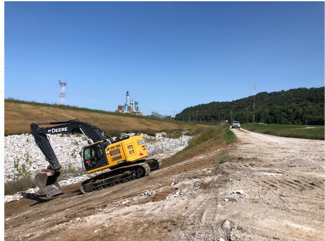
Facing north along levee.
