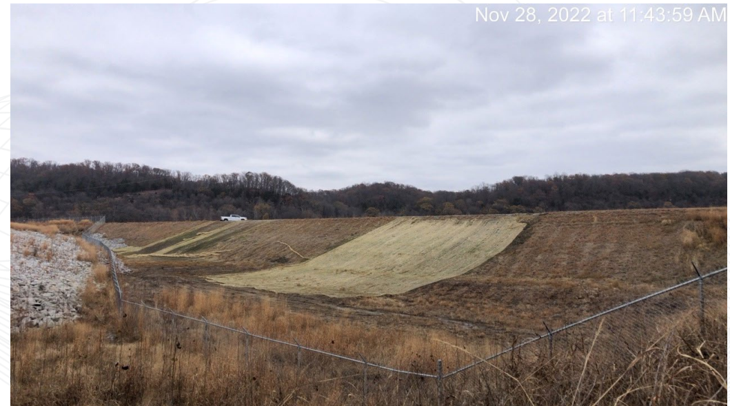
Facing northeast towards repaired section of USACE levee.
