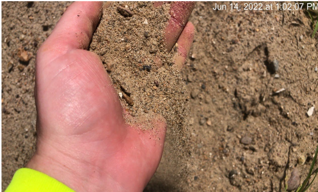
Close-up of exposed GTEC levee material.
