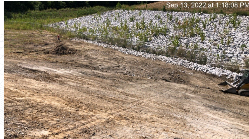
Facing southwest towards impoundment cap – repairs of fence undermining, levee, and riprap visible.
