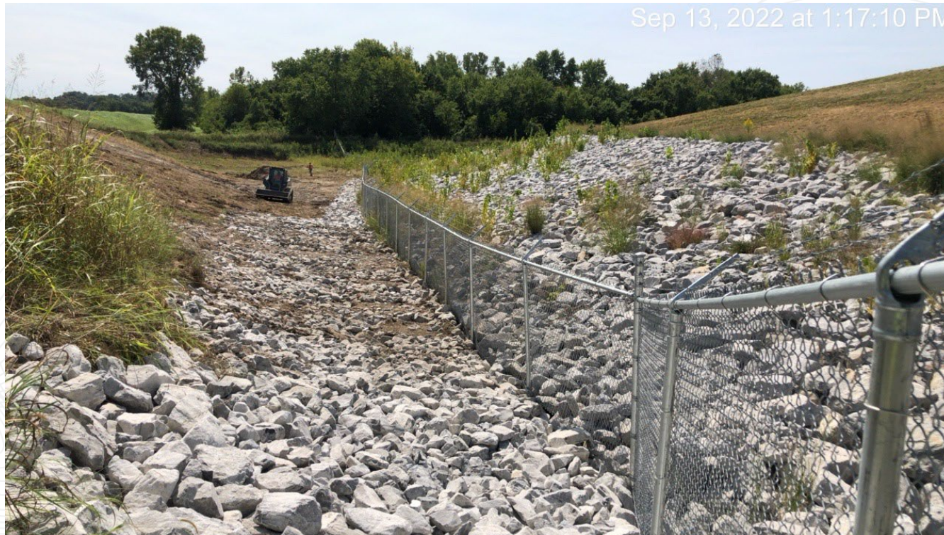
Facing south along recently repaired fenceline area.
