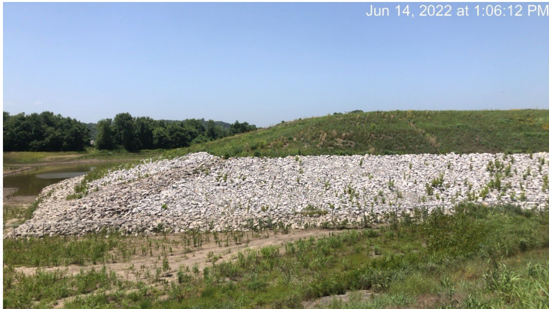
Looking west from Army Corps of Engineers Levee.
