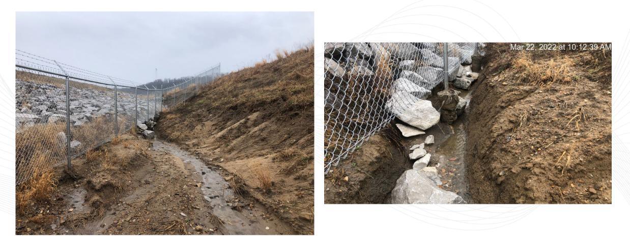
Fence undermining and GTEC levee erosion on SE side of closed CCR impoundment cap.
