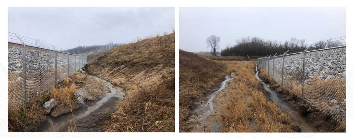
GTEC levee erosion and riprap undermining on SE side of closed CCR impoundment cap.
