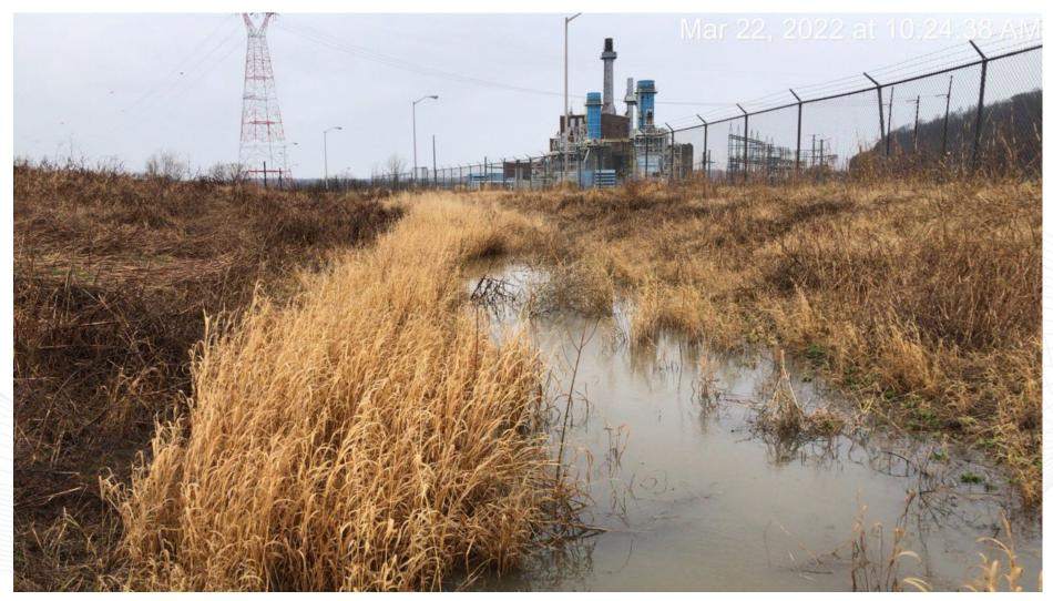
Ponding on NE side of closed CCR impoundment cap along GTEC levee (looking south).
