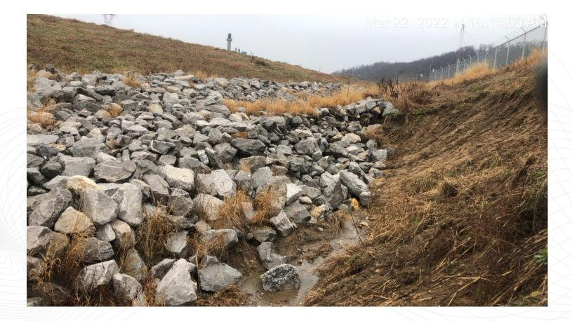
Ponding on NE side of closed CCR impoundment cap along GTEC levee (looking north).
